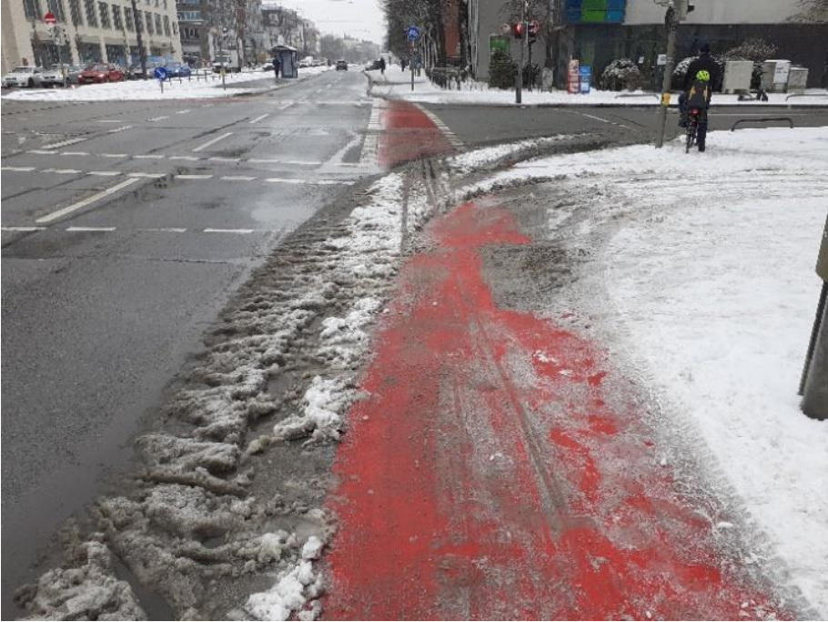
Fig. 4 - Snow bulge at crossing section [picture source Wiesler, 2022]
