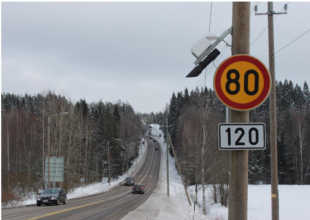
Figure 1. The compact road weather station installed on a wooden street light pole. The cabinet is on the other side of the pole at the height of the traffic signs.
