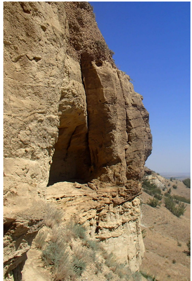
Fig. 9 Fractured rock spur next to the entrance to cave 6 (picture as part of the field survey in 2019) with two slope-parallel fractures. For comparison, the brownish weathered part is about two meters in height
