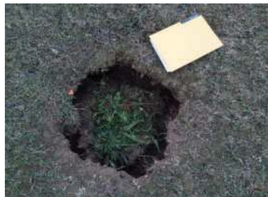
Fig. 2. The same sinkhole as in Fig. 1 . (identified by UAV) occurred in April 2018 (photo by R. Kanopienė).
