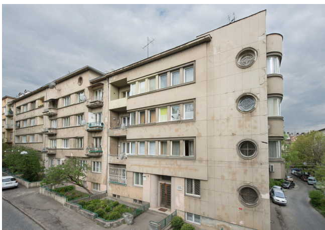
Fig. 10: Residential building in Sykstuska St. (today Doroshenko St.) 51. Architect: Jakob Menker, 1938/39.
