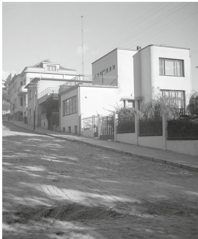
Fig. 8: A residential building owned by businessman Jonas Glemža on V. M. Putino Street, architect Jakovas Peras, 1936. Photo: Vytautas Augustinas, c. 1937, Lithuanian National Museum.
