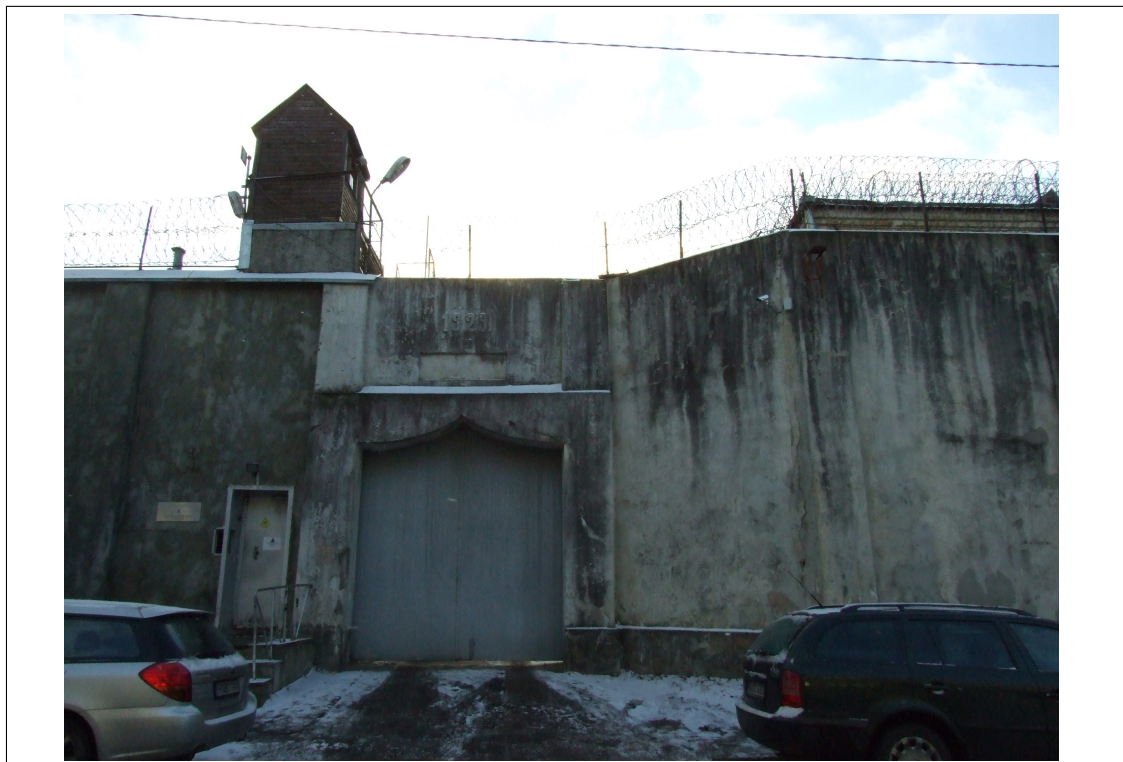
Figure 9: Prison hospital wall: no-one sees in, no-one sees out.
