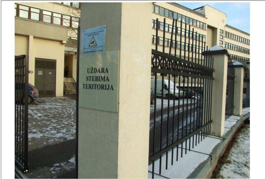
Figure 11: Ministry of Finance, backyard view: closed territory, warnings intact.
