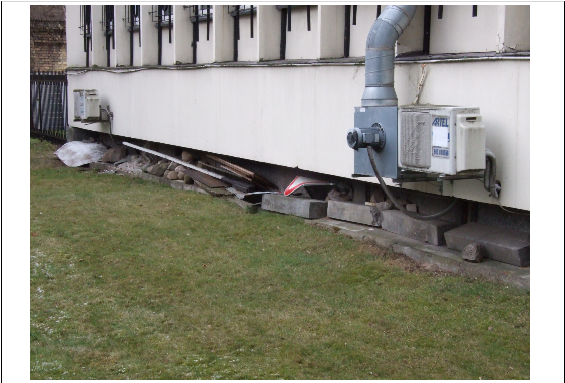
Figure 4: A traffic sign in the foundations of the supreme court.
