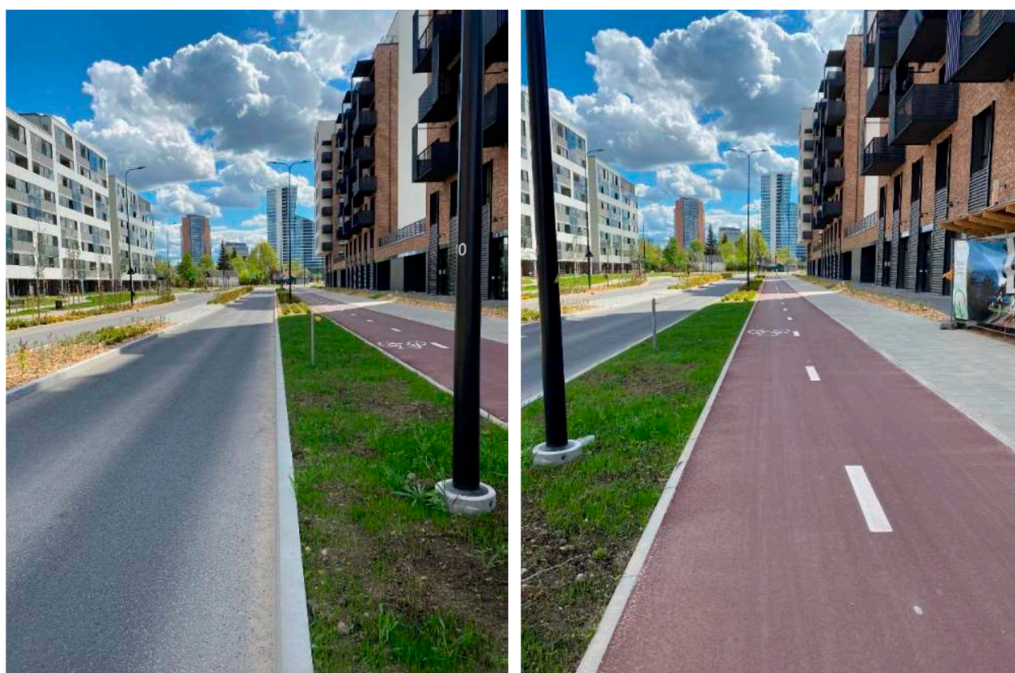
Figure 2. The first research object, the carriageway (on the left) and the bicycle path (on the right) on Kernaves street in Vilnius city.
