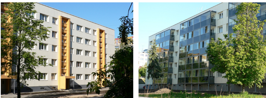
Fig. 8. Experimental upgrade project of a 5-story panel apartment building in Žirmūnai. Photo of the main entrance and yard facades [photo by Danas Ruseckas, 2004].
