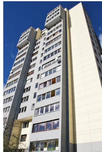
Fig. 9. Residential concrete towers in Lazdynai. On the left: the variety of upgrade styles and levels [photo by Bronius Jablonskas, 2020]; on the right – upgrade with ventilated façade ignoring the rounded elements [photo by Aušra Černauskienė, 2019].
