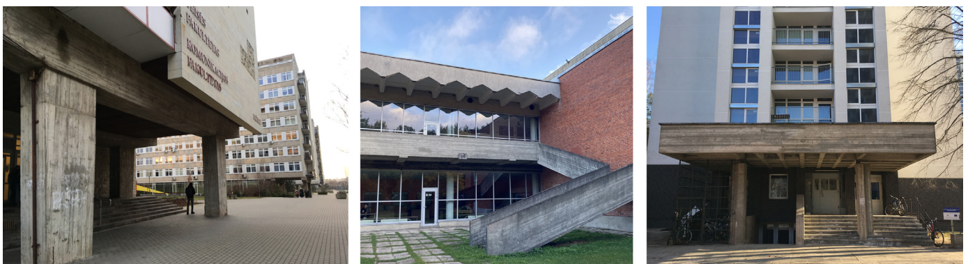
Fig. 2. From the left: Vilnius University (VU) complex from the side of the pedestrian alley; in the middle – VU connecting volume from the inner yard; on the right – entrance to the student dormitory [photos by Aušra Černauskienė, 2021–2023].
