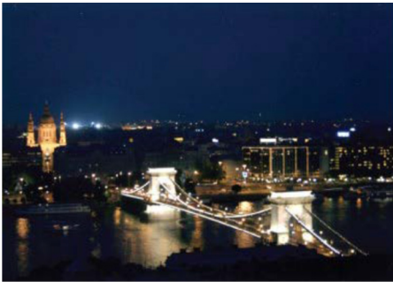
Fig. 3. Budapest at night. Bridge over the Danube River connecting Buda and Pest. The cables between the two main supports are in the shape close to the catenary. Photo: M. Sapagovas.
