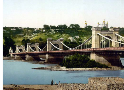
Fig. 4. The Nicholas Chain Bridge in Kyiv, circa 1900.
