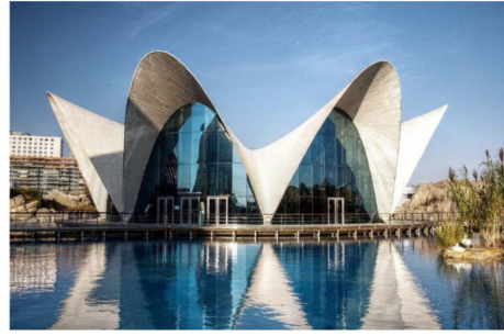
Fig. 13. Six-leaf clover-shaped minimal surface building in Valencia “Valencia L’Oceanogràfic”, the underwater restaurant. Architect F. Candela. Photo: F. Galbaldón, 2010.
