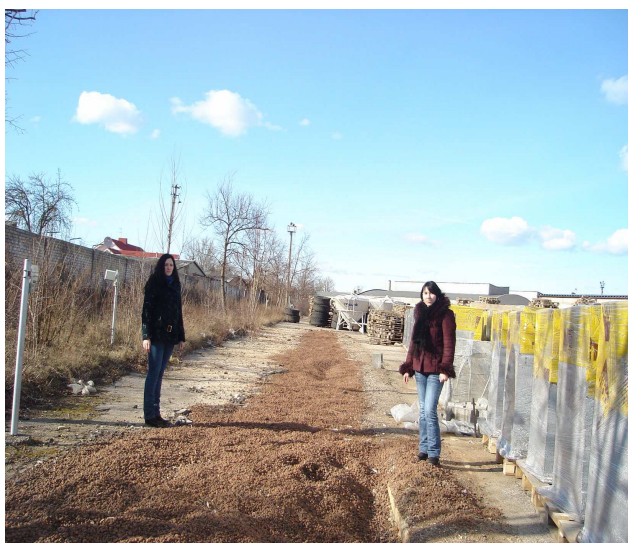
Fig. 3. A general view of vibroacoustical seams after implementation
