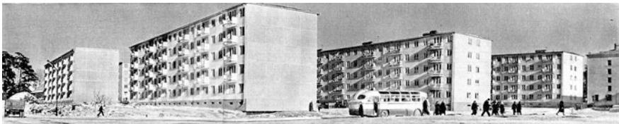
Fig. 4.2 The first prefabricated large-panel buildings (series) built in Vilnius in 1959. Source Naujoji tarybų Lietuvos architektūra (New Architecture of Soviet Lithuania) (1964). Vilnius: Mintis, p. 4
