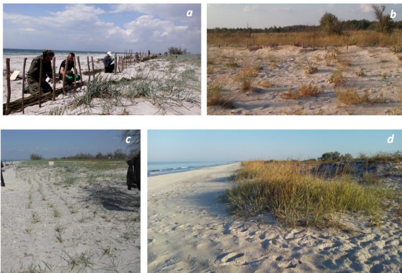
Fig. 2. Artificial strengthening and restoration of aeolian landforms within the frontal part of the Kinburn Spit: a – creation of a wind-damping shield (2013); b – the condition of the shield after five years; c – planting seedlings (2013); d – condition of the fixed area after five years.
